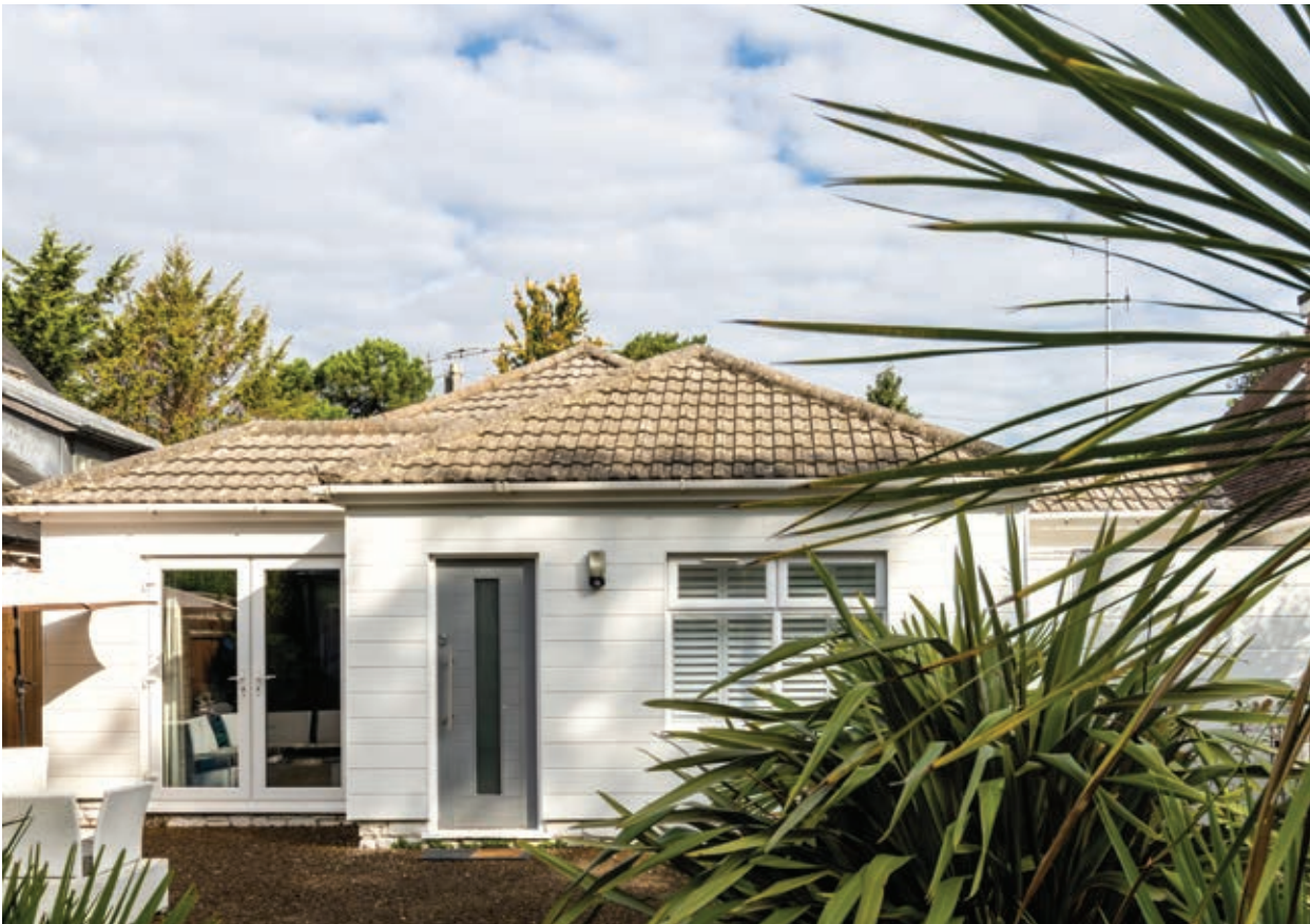
HardiePlank® VL cladding installed horizontally - Colour: Arctic White
